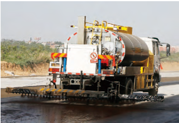
Bitumen spraying operation on surface of city road (automatic control)
