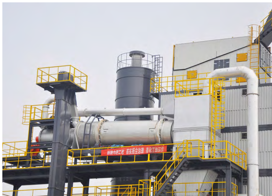
JNW4000 📍 China 🚚 320T/H 320t/h Advanced asphalt plant with RAP recycling (80t/h) in Henan Province. The 600t/h wet mix plant also made by ACE Group.
